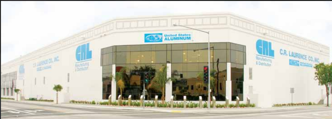
The New U.S. Aluminum Facility in Los Angeles, California
